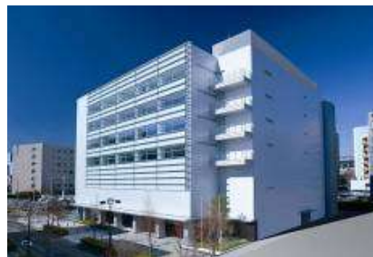
R&D Center and Head Quarters at Shin-yokohama
